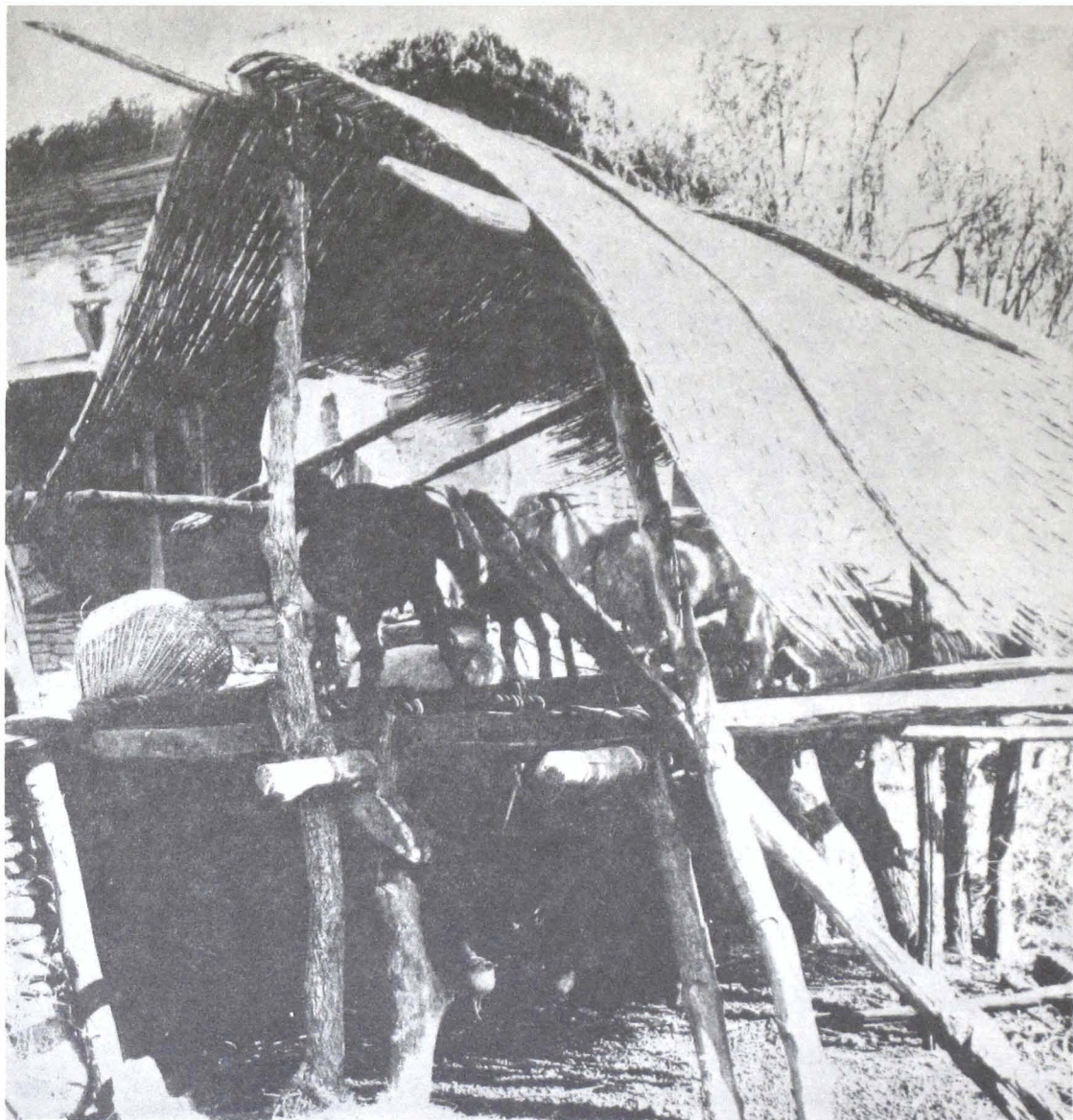
Fig. 21: Goathouse in the settlement of Gastkarker in the Thulo Khola. The roof shows the common construction with ridge-poles, ridgepurlin, and pillars. The goats are kept on a platform of round beams between which the excrements fall through, the floor thereby remaining tidy. (14. 1. 1977, photo : M. Kuhle)
