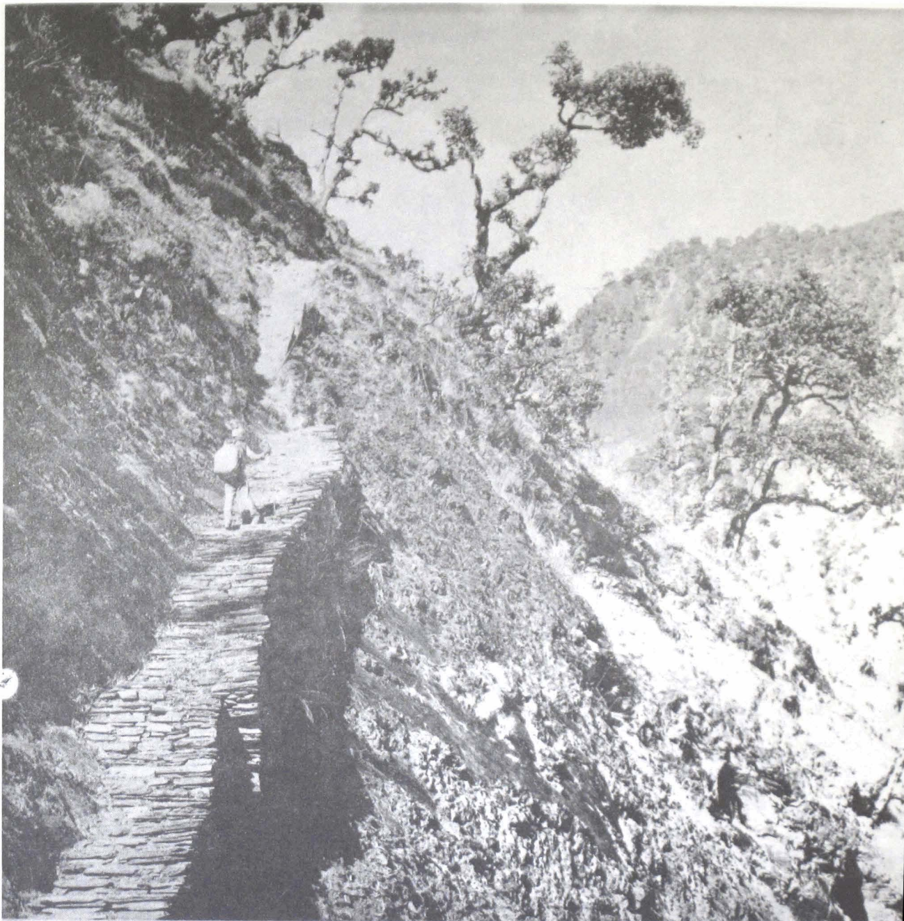
Fig.13: The trade road branching off from the Mayangdi Khola and ascending the Dhola Khola; here between Nerbang and Arche, from where it goes on to Gurjakhani. At this point, 2000m above sea-level, the road is traced alongside a smooth slate wall with the help of elaborate artificial constructions. The steps are slabs of cut slate. The evergreen trees along the road have been lopped for live-stock fodder. (29.1.1977, photo: M. Kuhle)
