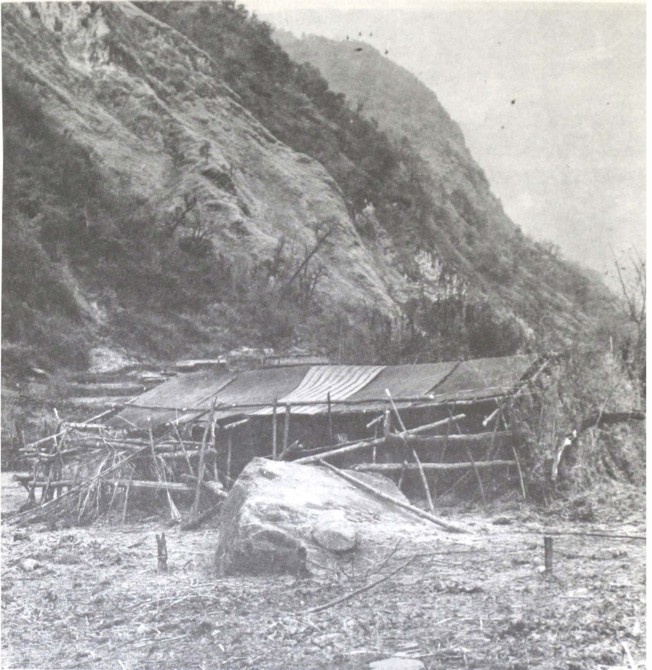
Fig. 19: Shed for water buffalo in the settlement of Fedi in the Thulo Khola, 2170 m above sea-level. The roof consists of bamboo matting, the gable fronts being enclosed with bamboo. Several wooden stems form a row of ridgepoles in whose forks several ridgepurlins are held. Several upright posts hold the struts that extend from them. The shed is open at the broader side. (11. 1. 1977, photo : M. Kuhle)
