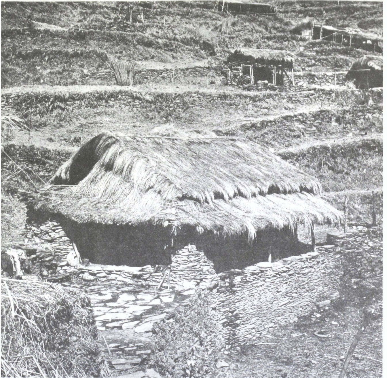
Fig: 20: Small house from the settlement of Bagara in the Mayangdi Khola, 2160 m above sea-level. This one-storey house has a grass roof and lean-to roof attached to the gable side which, like the loggia at the longer side, is covered with grass. The roofs of the loggia are supported by corner pillars of masonry as well as by wooden posts. In the background is a shed for firewood. (20. 1. 1977, photo : M. Kuhle)
