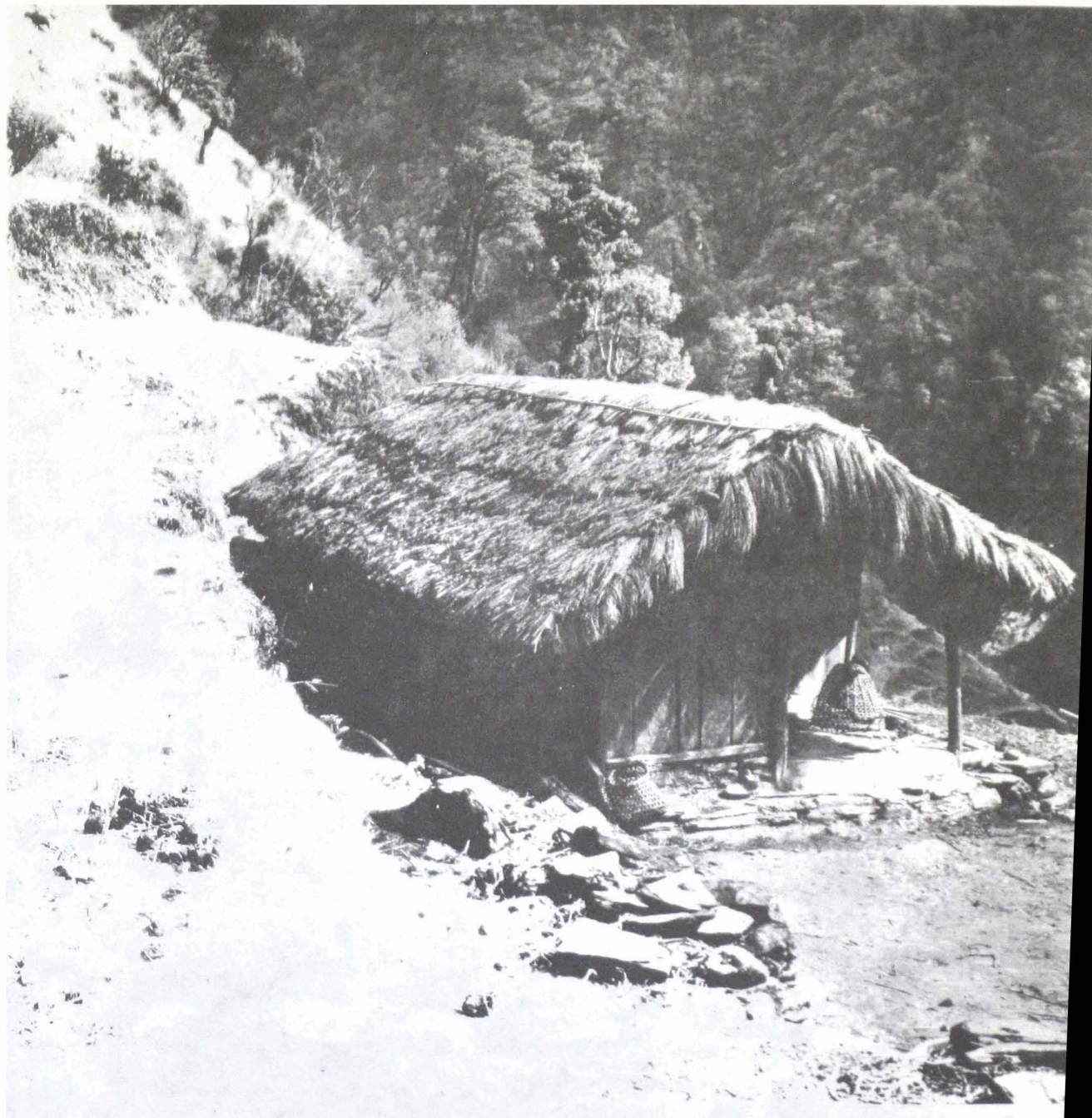
Fig.17: A small, one-storey house in the scatter settlement of Bagara in the Mayangdi Khola, 2150 m above sea-level. The roof is covered with grass, the walls are erected from vertical planks in the manner of a stockade. They rest upon a flat foundation of masonry. The house has a corner porch. (20.1.1977, photo: M. Kuhle)
