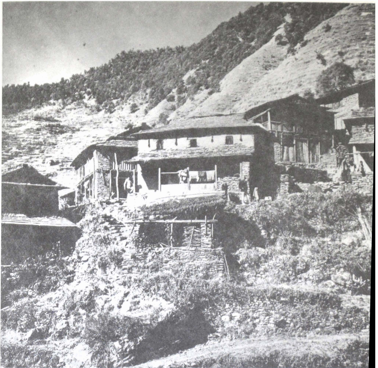
Fig.15: Close-up of the settlement of Malkabang in the Marang Khola situated about 2100 m above sea-level. Buildings are both daubed with loam and left undaubed. There are loggias on one side, but also loggias surrounding the entire house, sometimes one-, sometimes two- storeys high. The surrounding two-storey loggias form a second outer wall for the house. Loggias are often closed-in with wooden planks (cf. right). In the background the transition from fields to woods can be seen, the latter extensively degraded by use as pasture. (16. 1. 1977, photo: M. Kuhle)
