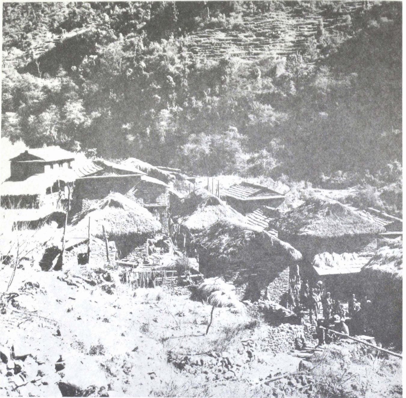
Fig.14: Detail photograph of the settlement of Gastkarker in the Thulo Khola 2000 m above sea-level. We find a combination of diverse roof forms: comparatively flat slate roofs, steeper grass and thatched roofs with and without hips, thatched roofs with slated loggia or vice-versa. The high-built ridge is conspicuous on the slated roofs. Lean-to roofs are only attached to slated roofs. (14. 1. 1977, photo: M. Kuhle)
