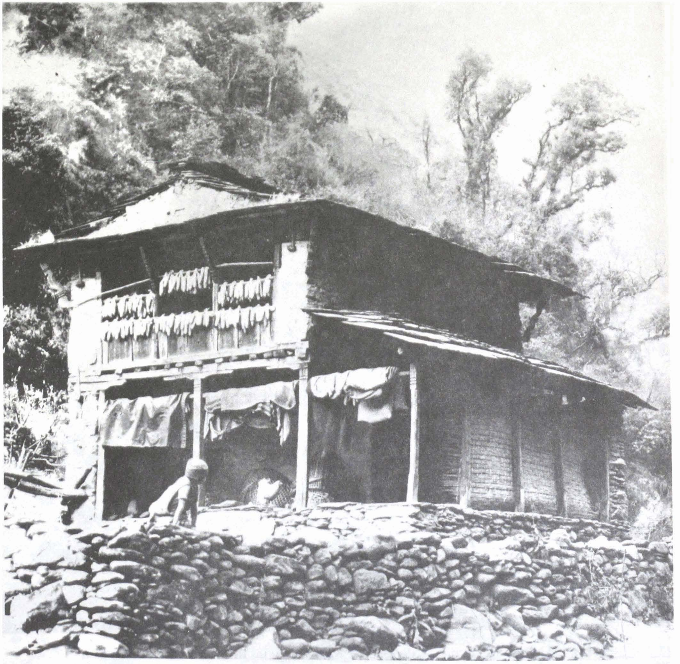
Fig.16: House of a single settlement in the Mayangdi Khola, 1560 m above sea-level. Here is a rare combination of loggias integrated into the outer walls as well as an attached loggia alongside with a lean-to roof. The function of the large window front in the upper storey for air circulation becomes apparent. Under shelter of the attached lean-to roof corncobs are being dried. (19.1.1977, photo: M. Kuhle)
